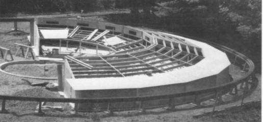
the edge of the slab extends beyond the walls so the wall sheathing cannot drop down past the top of the concrete as with most buildings. Ideally, the slab outside the walls should have a downward slope away from the building so water from the roof drains away from the mud sill.
