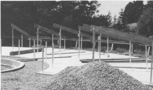
Aluminum columns are held in position by temporary supports as Jon Nagel (top, left) pours fast-setting grout to hold them permanently. GGLS members inspect the concrete after forms have been removed (top, right) and begin to locate the holes, just under the surface, where the columns will go and to drill for the bolts that will hold the mud sill. Note how close the front of the roundhouse is to the rim of the 14-foot turntable pit. This gives as much
