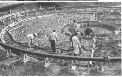
Dalt Bergstedt photographed Steve Booth (top) as he shoots preliminary levels for the new roundhouse. With no way to get the readymix trucks close to the site, concrete was pumped (center and below) for the roundhouse floor and turntable pit. Shortpieces of white PVC pipe are at the locations of the 44 columns to be grouted in later.
